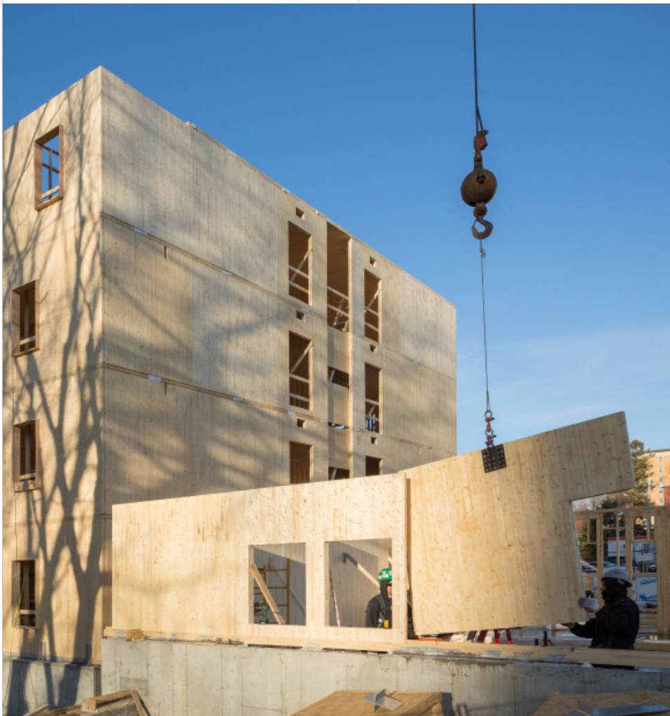
FIG 1: Open panel installation 70
